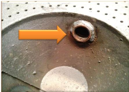
Cut in the hole in the fan sleeve which will perform the hole to pull the fireproof cable through.
