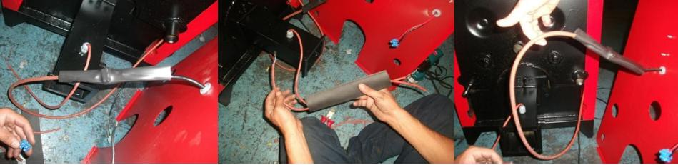
Connect the second outlet cable of the electrical power unit with the cable going to control panel of the boiler. Insulate the connecting socket tightly with fireproof insulation.
